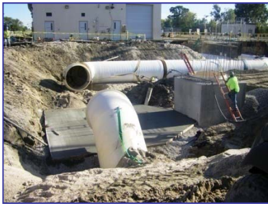
Construction of yard pipe at the SWWTP that will convey wastewater throughout the plant.
