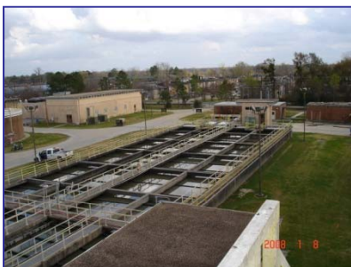
Design of the SWWTP Phase 1 project started in June 2008.
